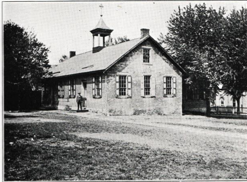
FORMER SCHOOL BUILDING on Northampton Street
