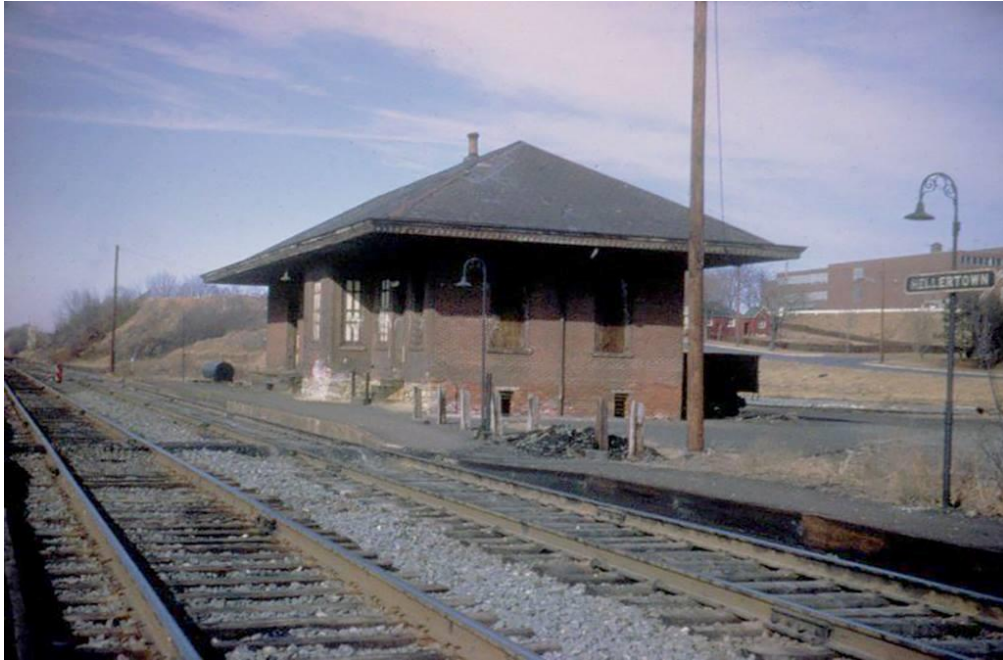
Photo of the Railroad Station Looking North in the early 1970's
