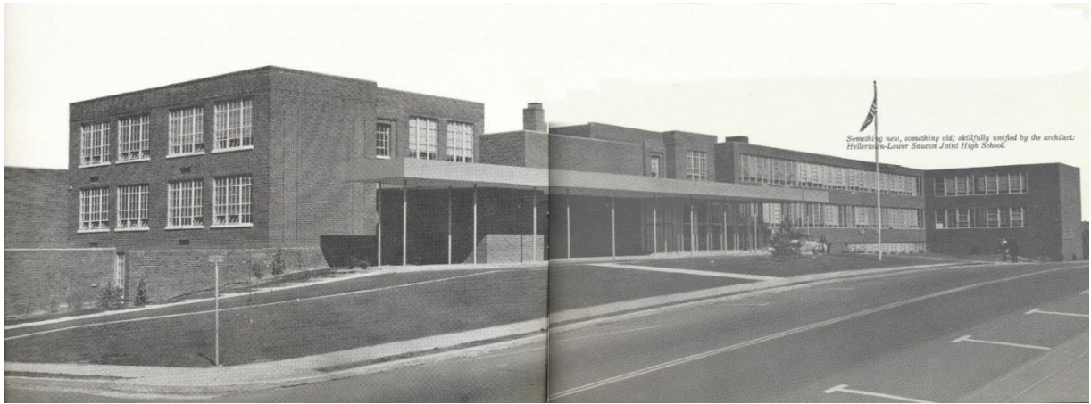
Overall View of the Entire School Building After Additions – Looking Northwest
