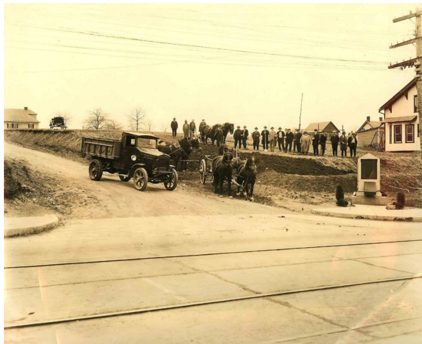
Ground-Breaking for the Legion Building April 22, 1926
