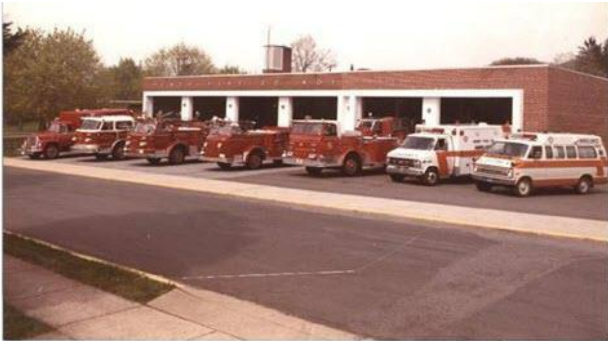
In the Late 1970's a Building Expansion Project Added Three More Garages as Additional Equipment Became a Necessity – October 1979
