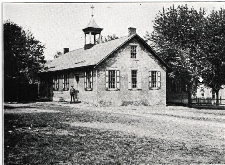
FORMER SCHOOL BUILDING on Northampton Street
