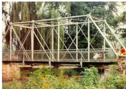
Walnut Street Bridge, 1970
