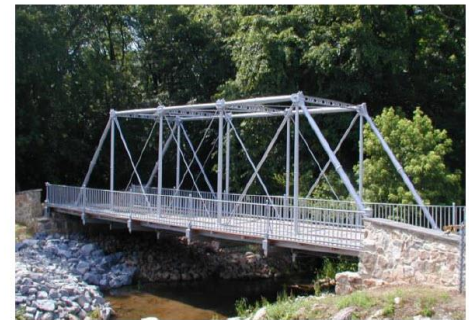
Walnut Street Bridge, 2000
