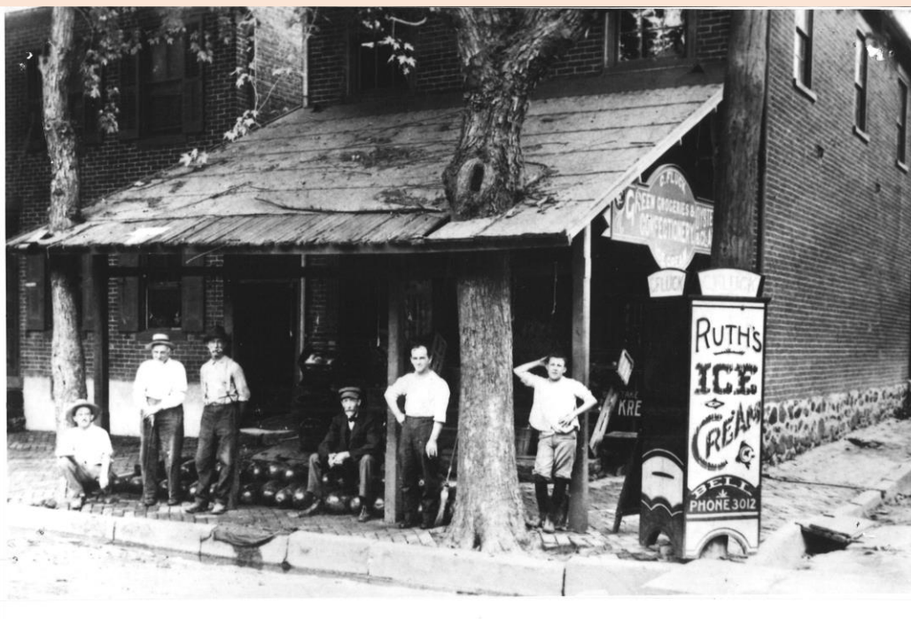
Calvin Fluck’s Green Grocery and Confectionary store at 612 Main Street circa early 1900’s before Main Street was paved in 1923-1925. Note the trees growing through the roof overhang. Today the Hellertown Bakery and True Shepherd Health Care L.L.C. both occupy this site.
