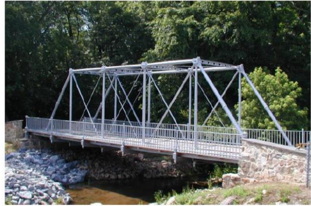
Walnut Street Bridge, 2000
