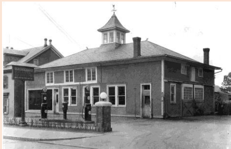
Geyer Auto Company c.1925 site now occupied by Lehigh Valley Health Network building
